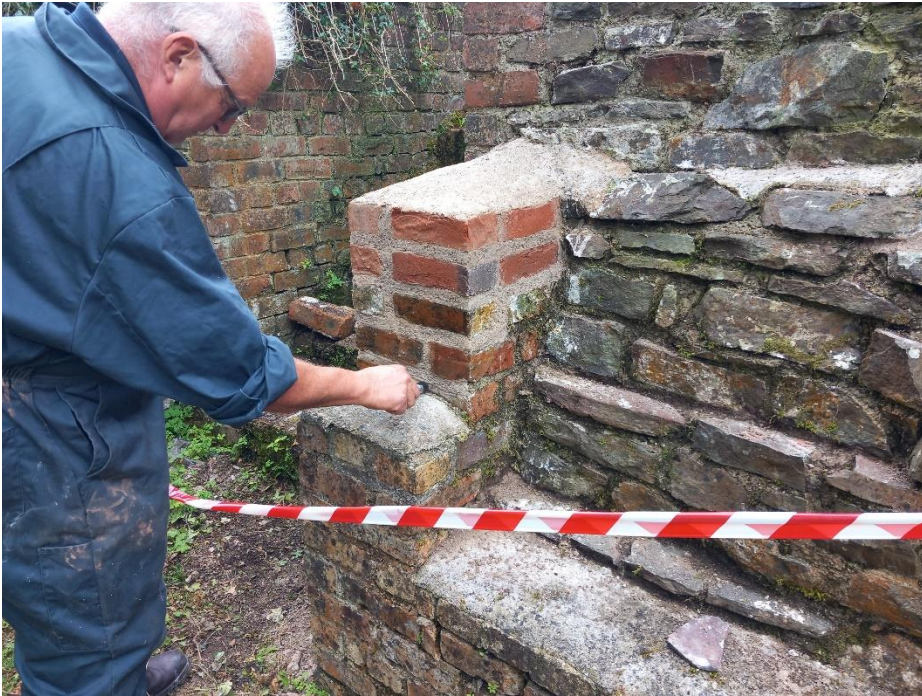
Dressing the mortar to repaired section of wall
