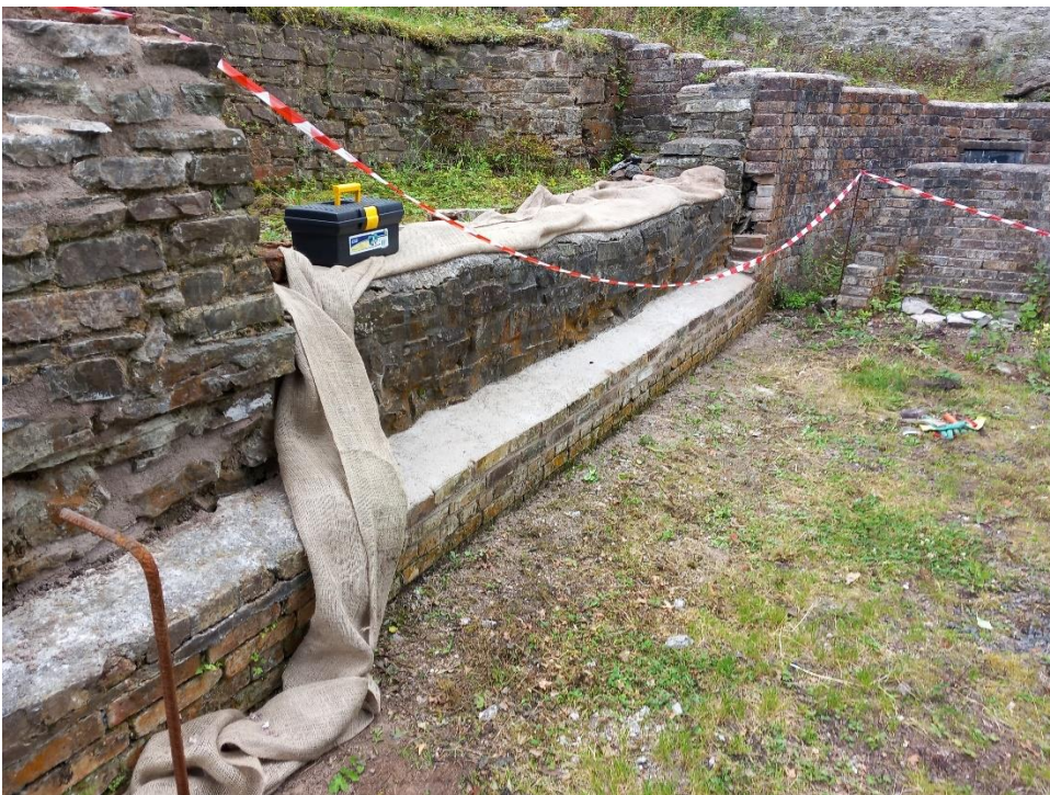
Completed stabilisation/repair to damaged wall
