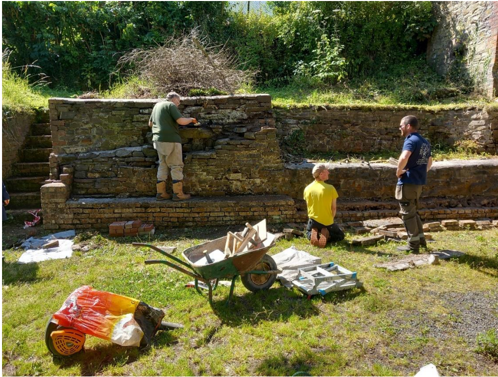
Reconstruction of lower wall and repointing upper wall
